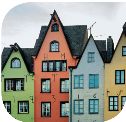
Waste heat recovery, Cologne
