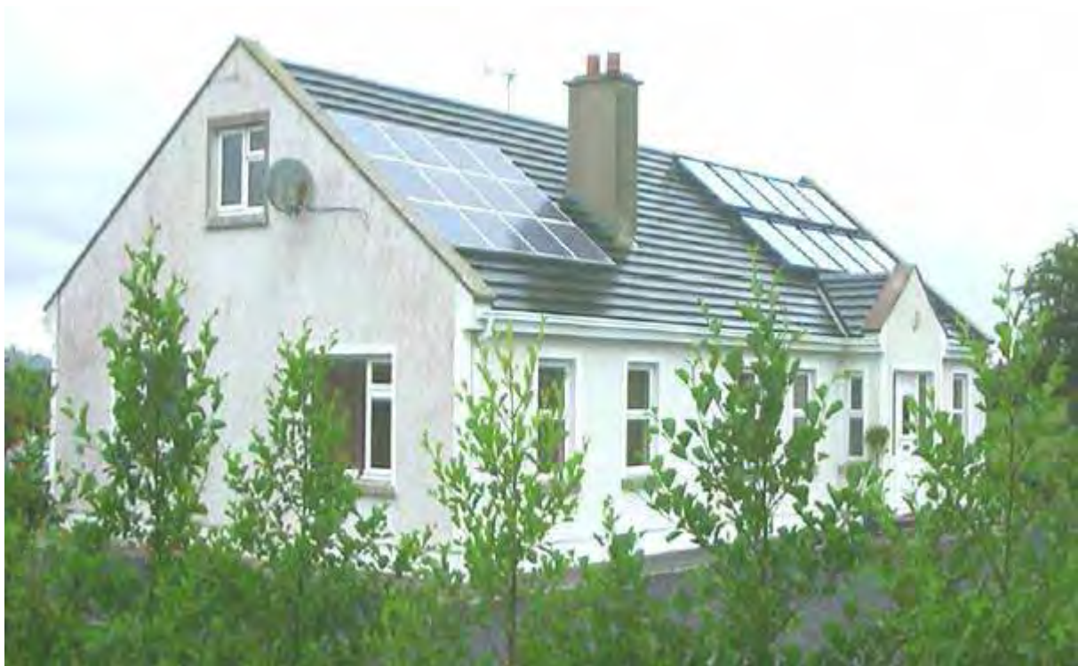
Figure 4-1: PV installation and Wind system for residential dwelling.
