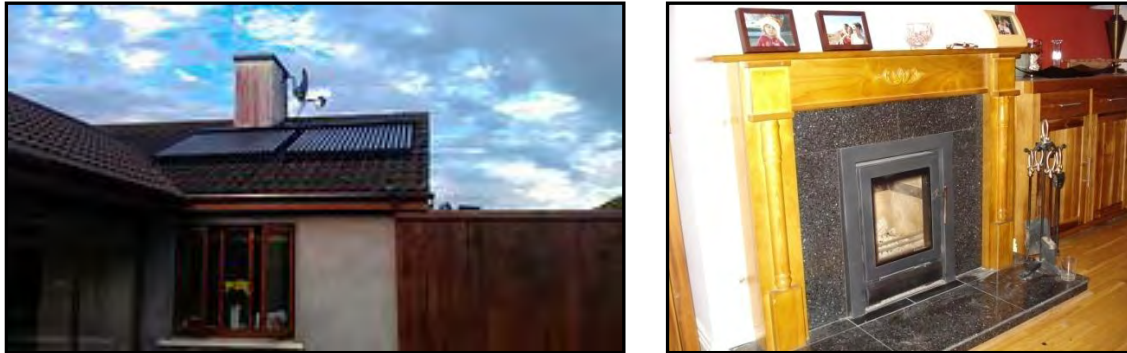
Figure 2-1: Sample installations (solar panels, wood stove insert)
