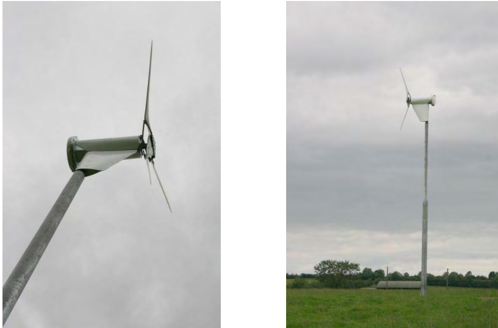
Figure 3-2: Micro Generation 6kW Wind turbine (Proven)
