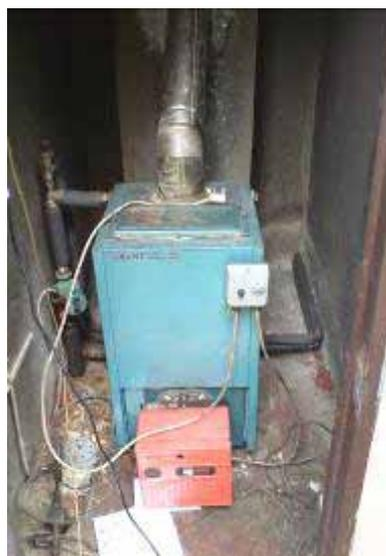
Figure 2-8: Typical Boiler Installation in Existing Dwelling
