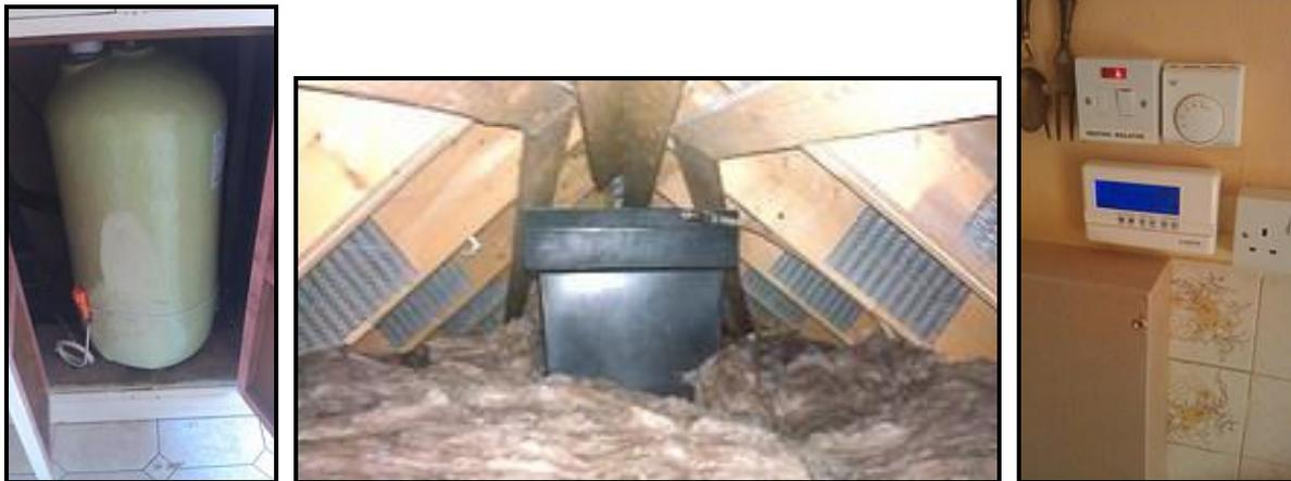
Figure 2-3: Sample Installations (Hot water Cylinder, Attic Insulation, Heating Controls)
