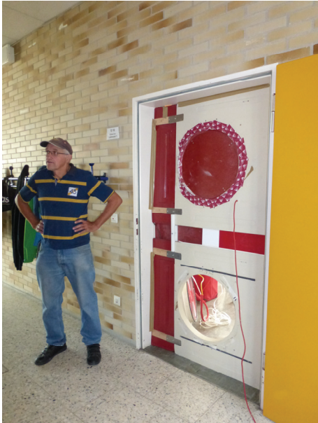
Figure 5: Blower-door test at the Solitude-Gymnasium, Stuttgart.
