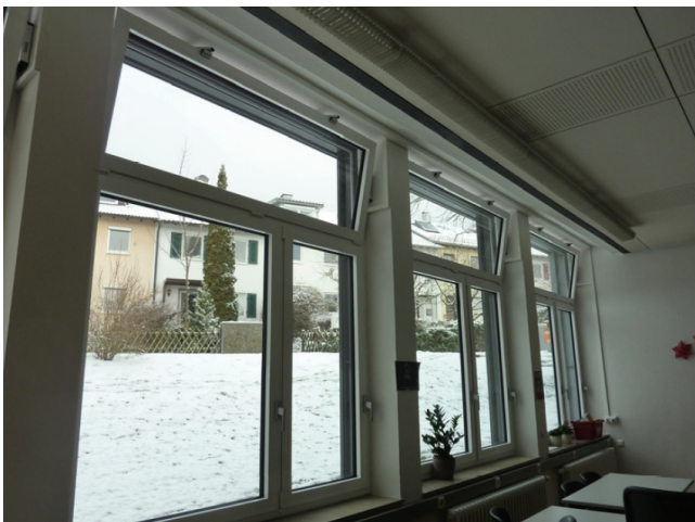
Figure 8: Windows with automated opening during breaks and manual switch for the teacher during classes.
