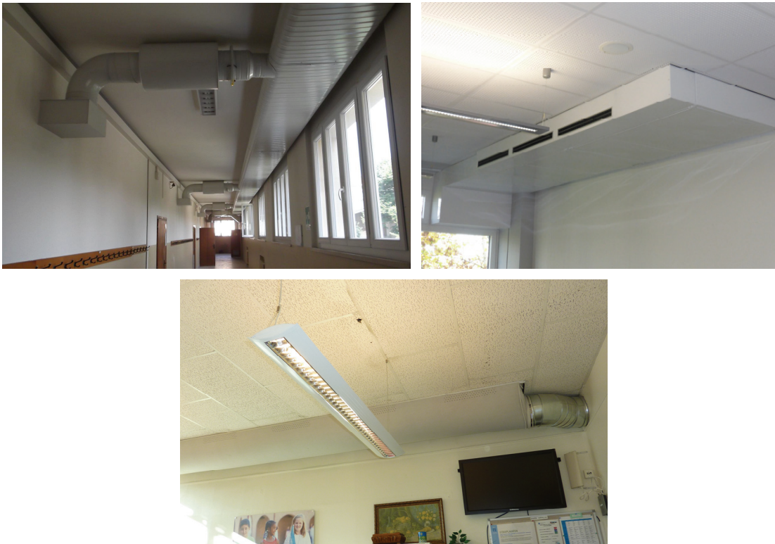
Figure 9: Ventilation systems used in the School of the Future case studies: Top left: decentral ventilation system for 4-5 classrooms (Tito Maccio Plauto School, Cesena). Top right: decentral ventilation system for a single classroom (Solitude Gymnasium, Stuttgart). Bottom: Supply system (distribution sail) in a classroom of the central ventilation system at the Brandengen School in Drammen.
