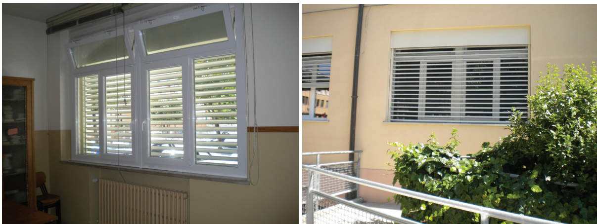
Figure 9: Security concept for night ventilation via overhead windows in the renovated Tito Maccio Plauto School in Cesena, Italy. Photo: M. Zinzi.
