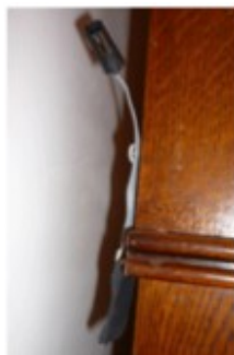
Figure 6 : Picture of a thermohygrometer installed in the back of a cabinet.
