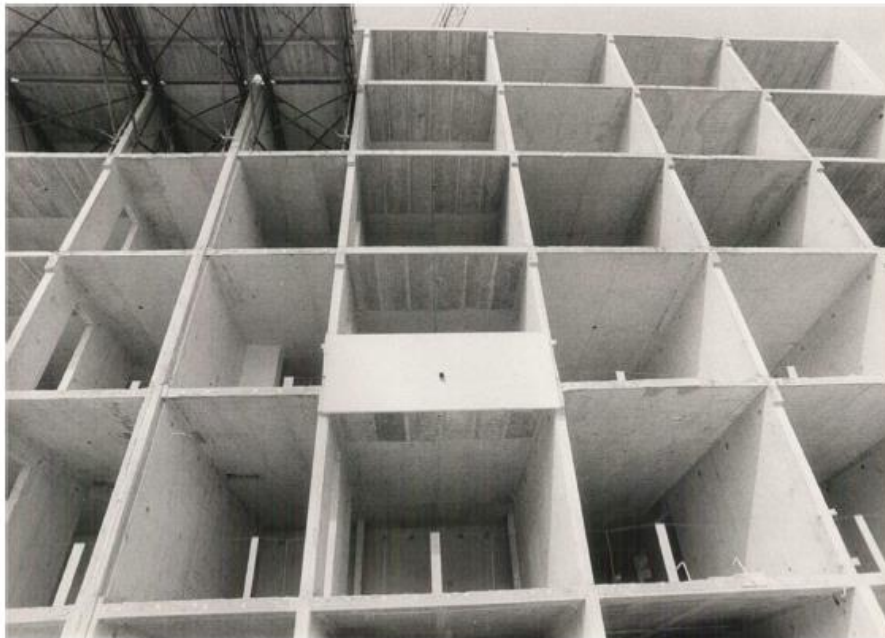
Figure 4: The Washing Machines, the "banches et tables" French constructive technique
