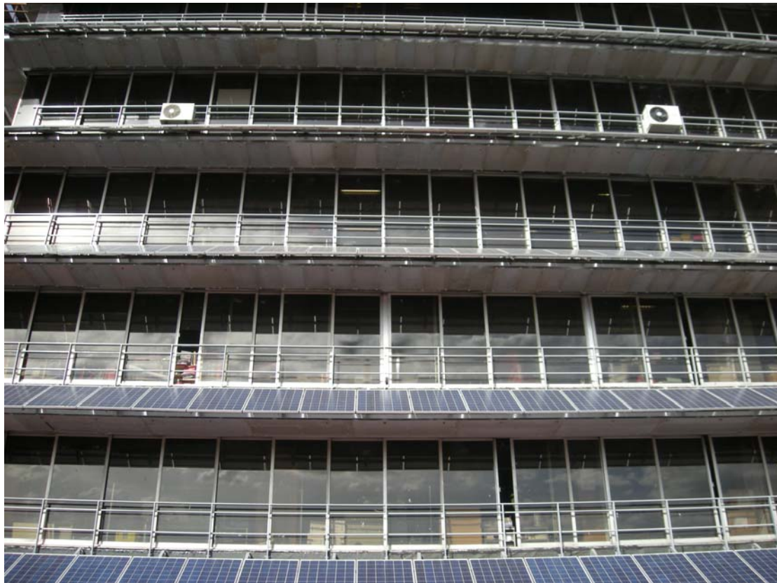
Figure 17 – PV panels on SW façade
