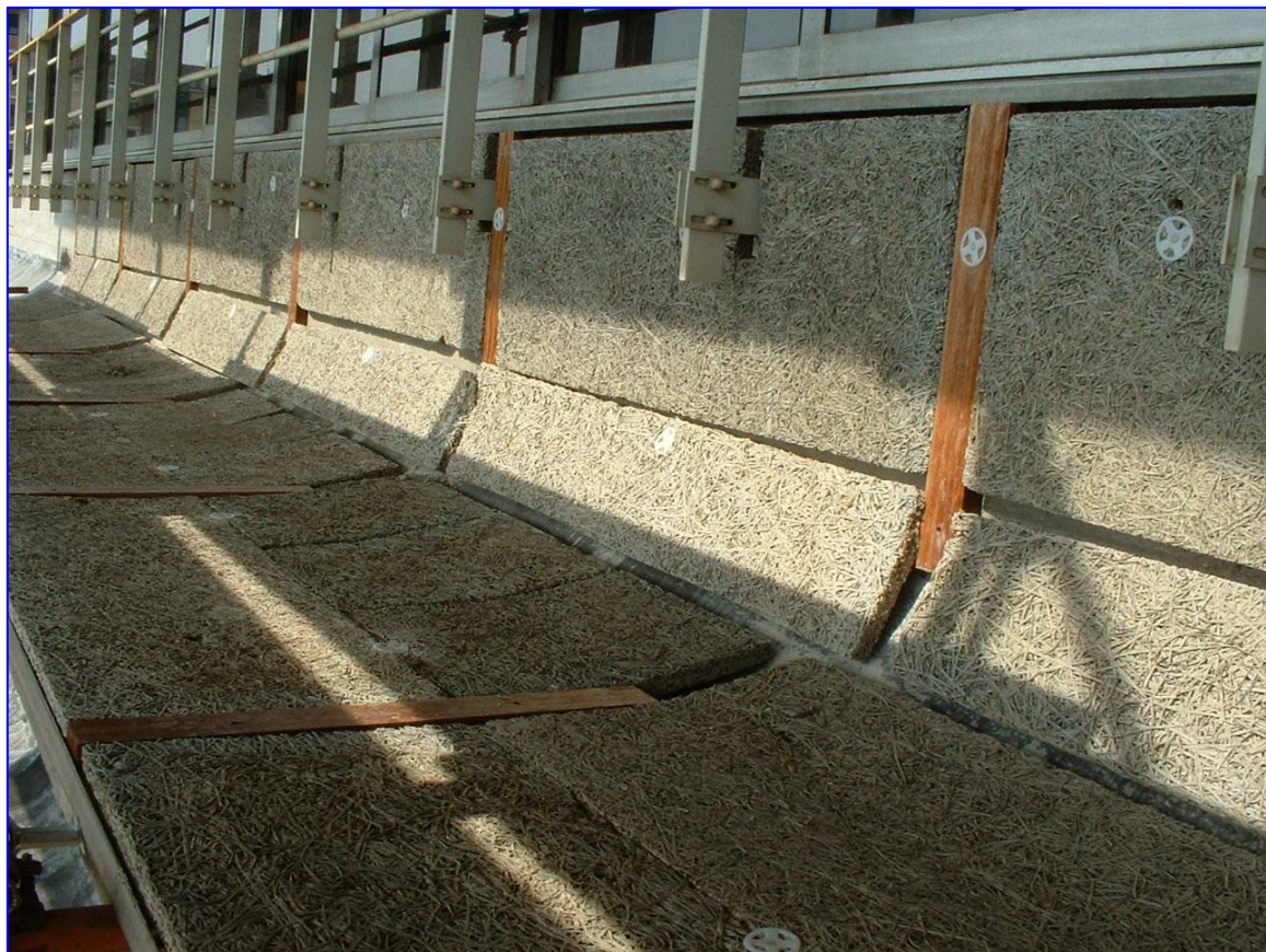
Figure 11 – Wood fibre panels posed over the overhangs' surface and walls
