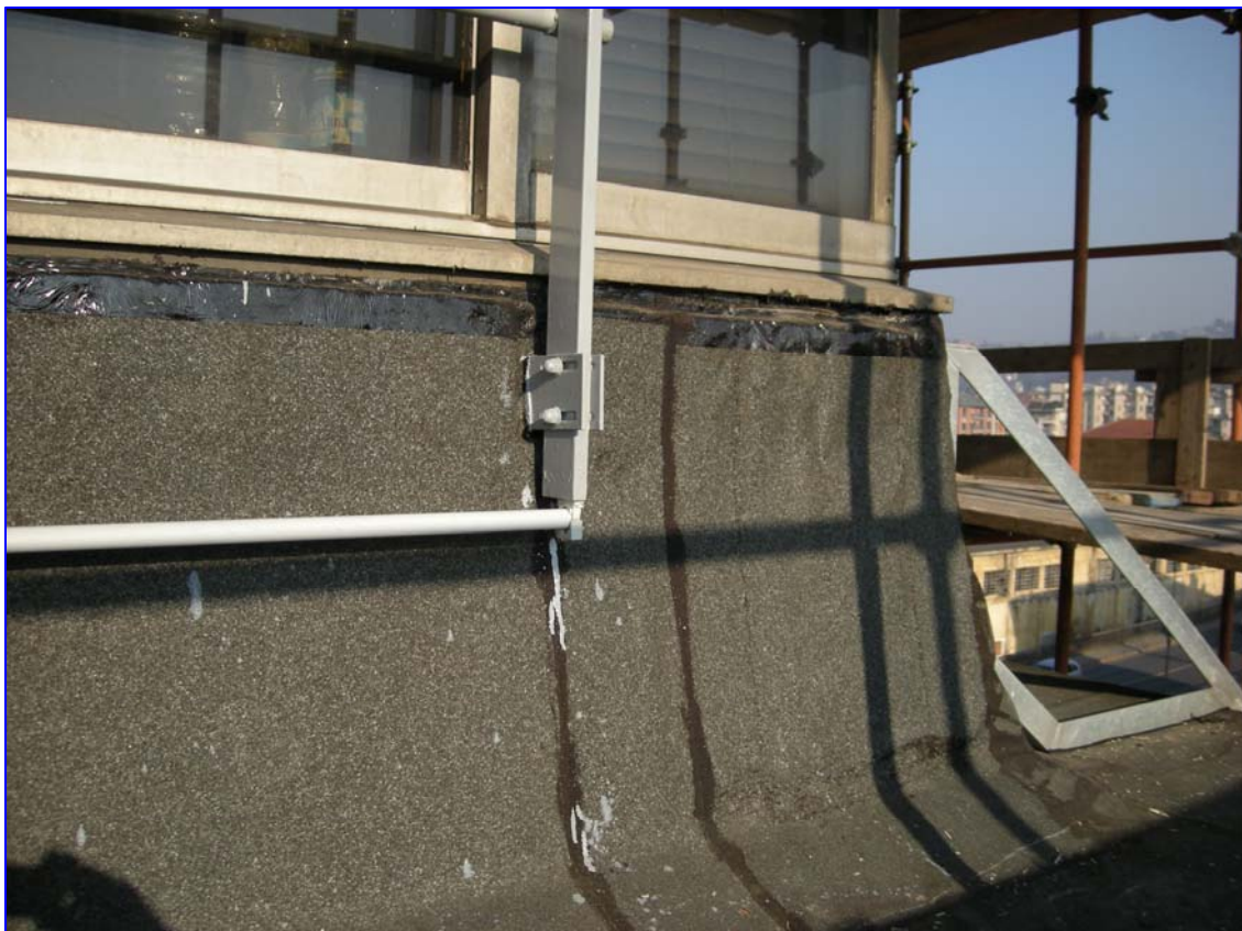
Figure 13 – The insulation completed with the bituminous sheet for rain shelter
