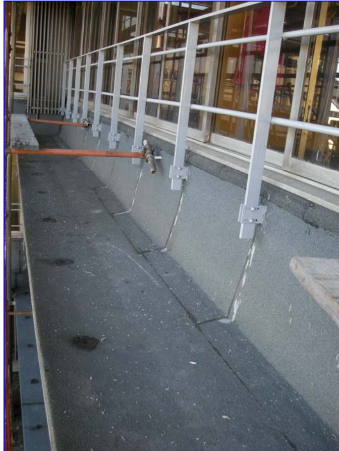
Figure 14 – The insulation completed with the bituminous sheet for rain shelter
