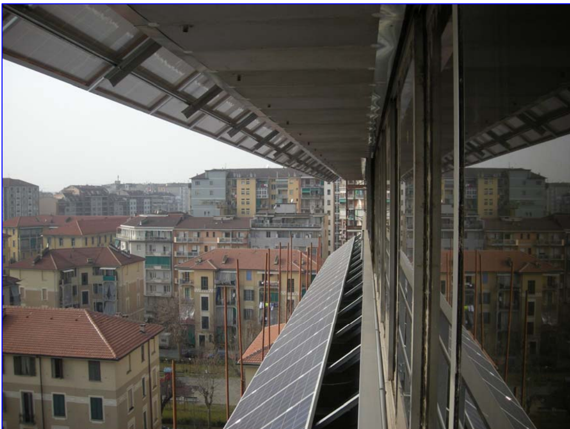
Figure 16 – Image showing the extension of the overhangs shape thanks to PV panels
