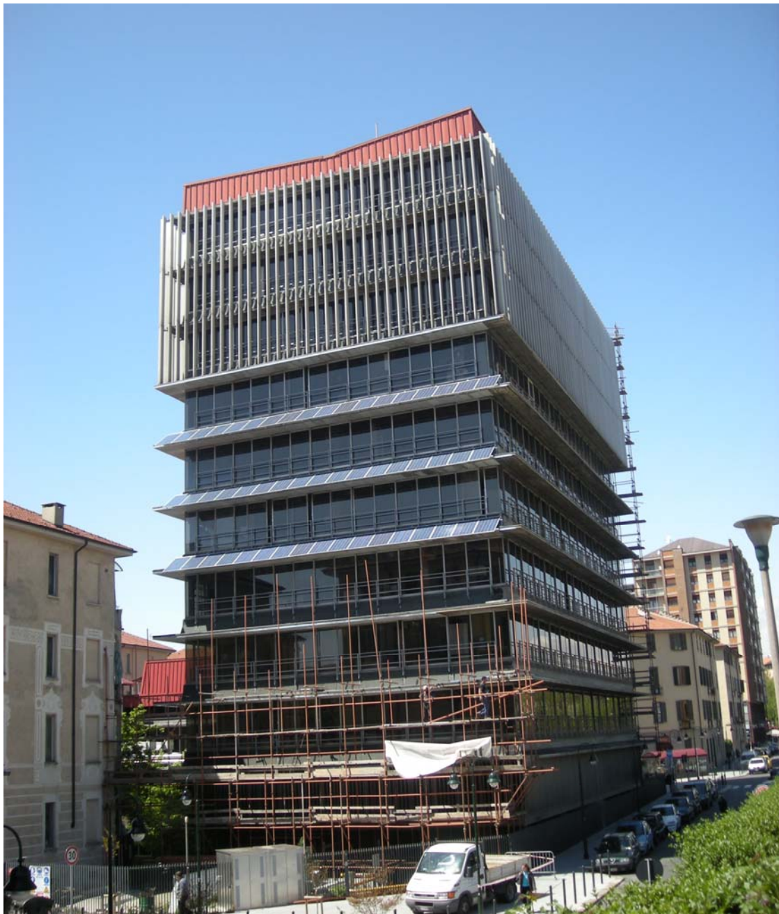
Figure 21 – PV panels on SE facade
