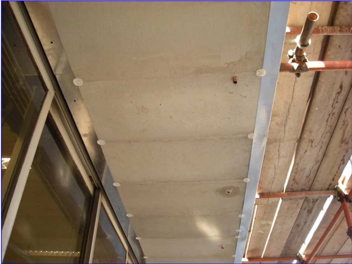
Figure 12 – insulating panels applied to the lower surfaces of the overhangs
