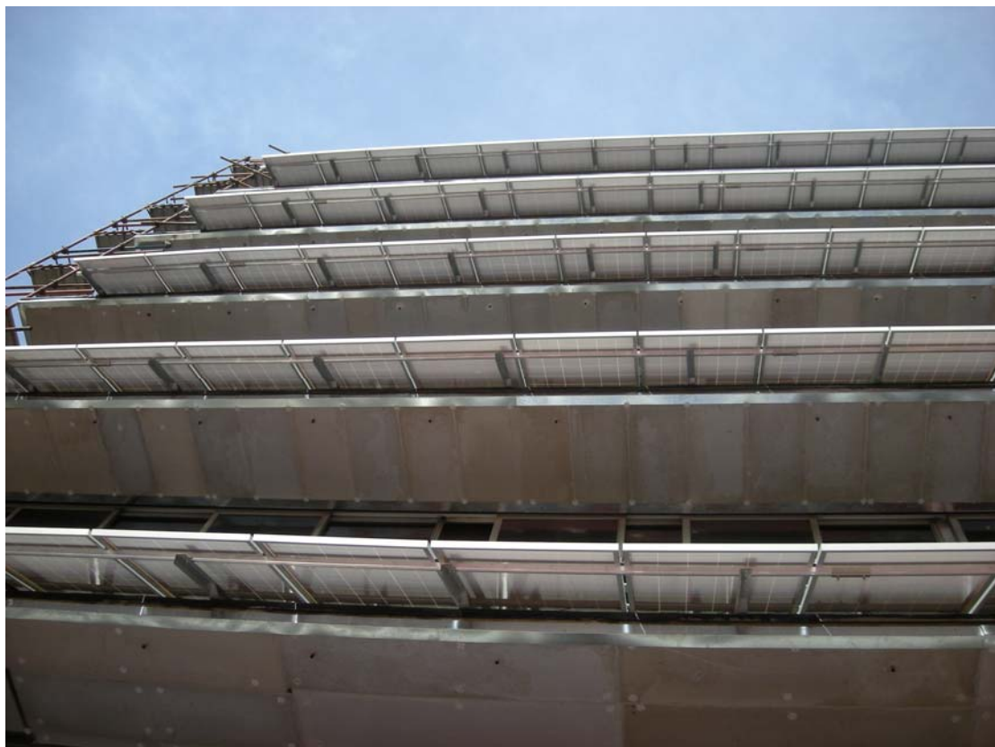
Figure 18 – PV panels on SW facade
