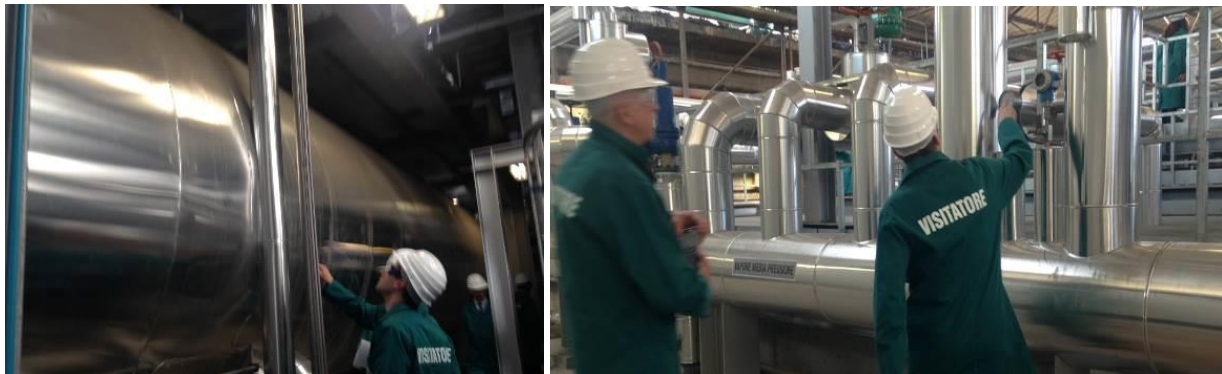
Figure 6. Steam Accumulator (left) and steam distributor (right). Source: Tecnalía
