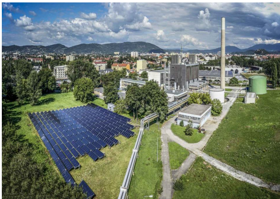
Figure 42. Aerial view of test field. Source: Solid.
