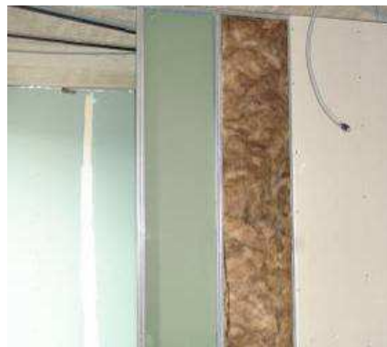
Partitions are being built. They consist of plasterboard – insulation – plasterboard fixed to an aluminium substructure. (March 2013)
