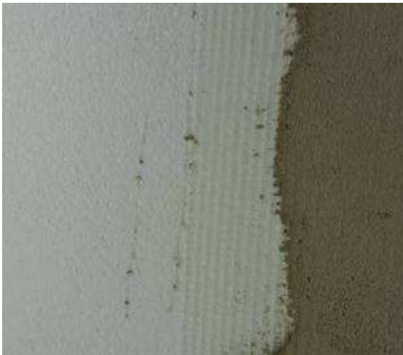
Fibre glass mesh and the application of the screed can be seen.
