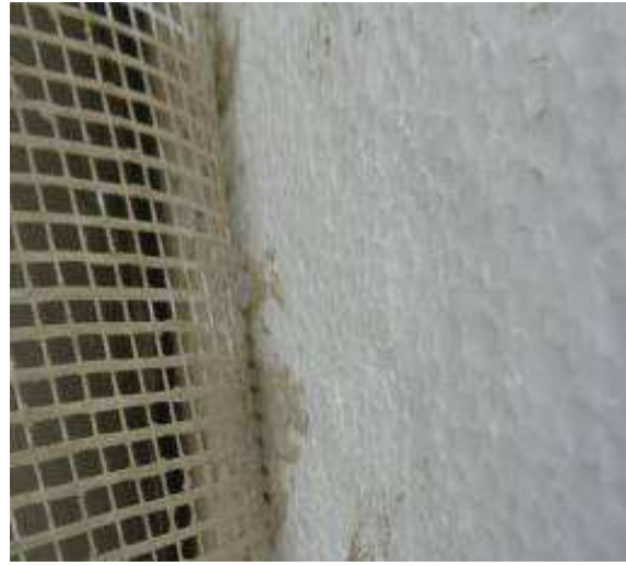
EPS and fibre glass mesh.
