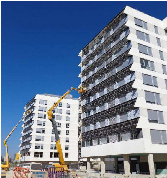
Façade insulation and structure for PV panels and enclosure beneath them.
