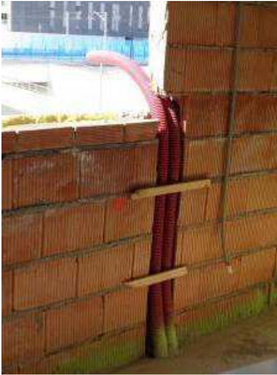
Tubes to carry the wires to the installations room.
