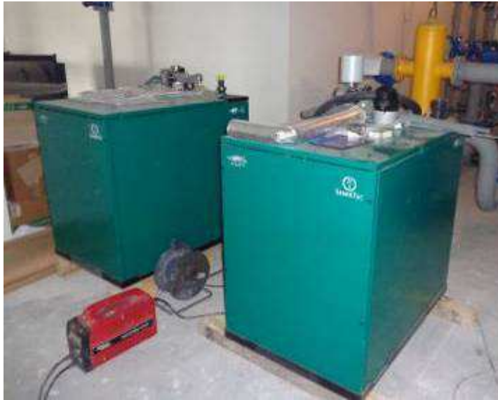
Micro CHP engines to be connected
