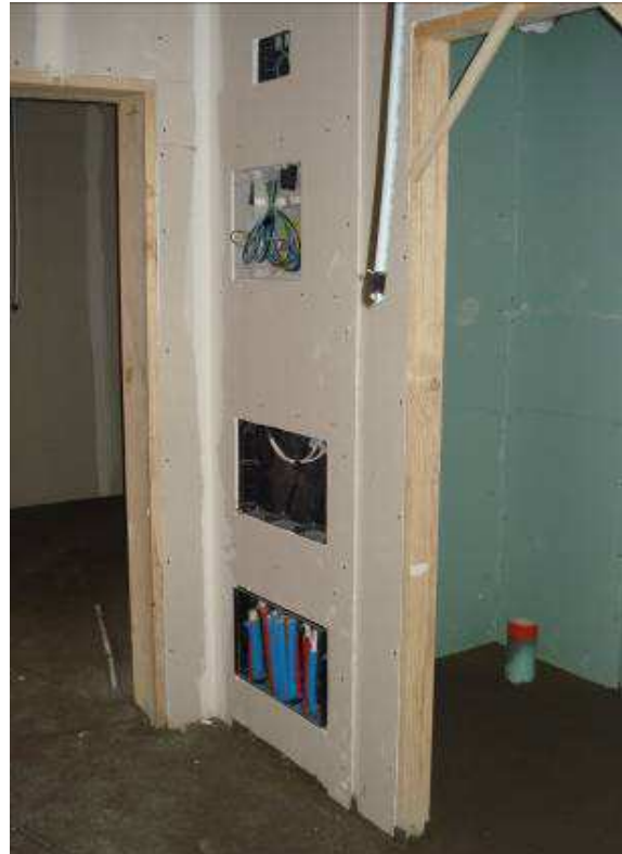
Screed over the floor before placing the flooring. Heating pipes run below it.
