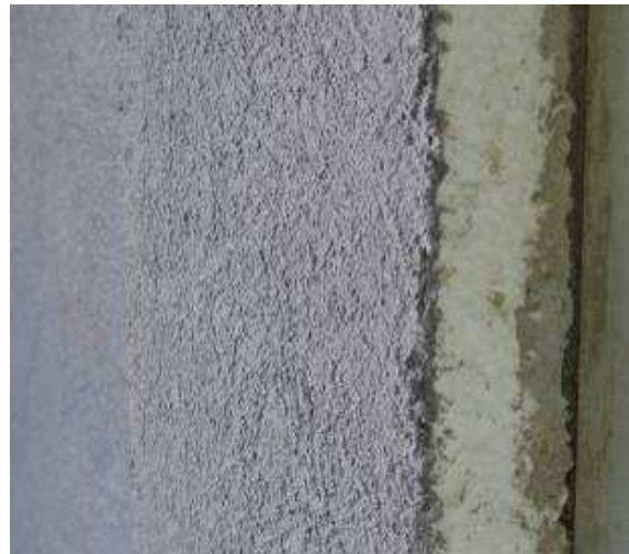
Fibre glass mesh and the application of the screed can be seen.
