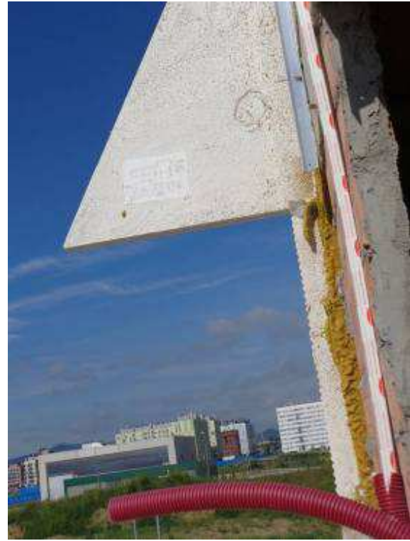
Channel for the wires and tube to carry the wires to the installations room.
