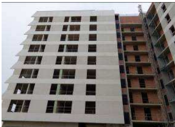
U shape East façade
