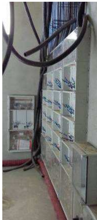
Installations register in each floor of the Electrical metering room. building.
