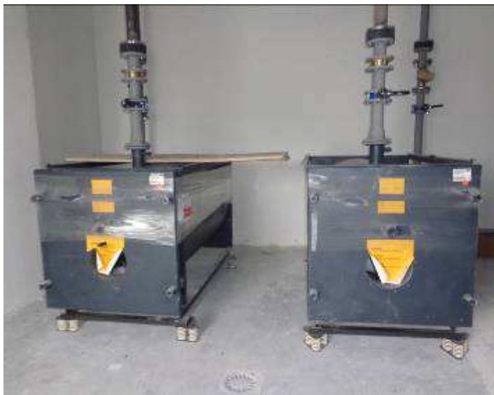
Condensation boilers to be connected to their chimneys.
