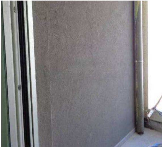
ETICS system in the balconies.
