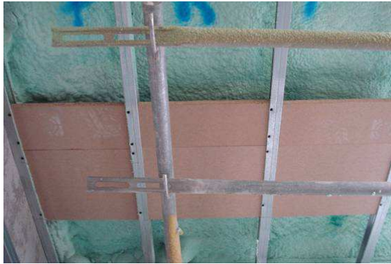
Substructure for the radiators. (November 2012)
