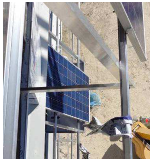
PV panels installation in a test mode.
