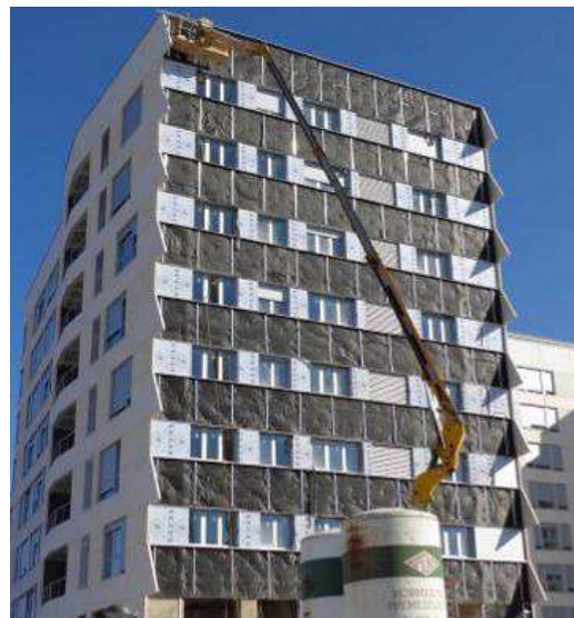
The insulation is set and after that PV panels and the enclosure beneath is put in place.
