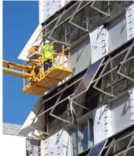
Façade insulation and structure for PV panels and enclosure beneath them.
