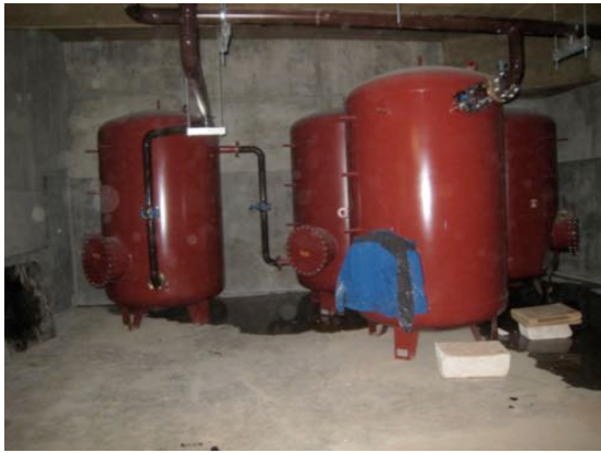
Figure 52 – Water tanks used as heat storage (December 2014)
