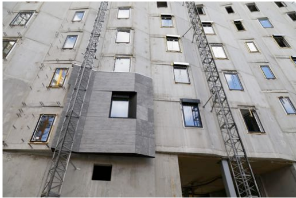
Figure 32 – Cladding of the northern façade of MINAMI (September 2014)
