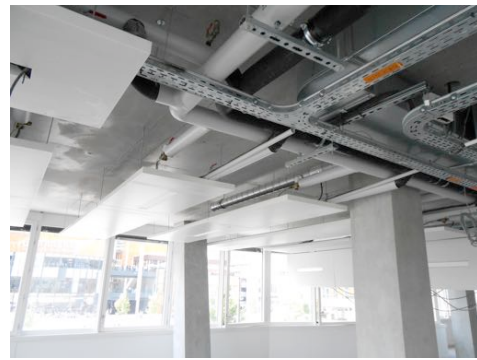
Figure 49 – Heat/cold ceiling emitters with LED light (July 2015)
