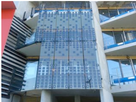
Figure 38 – Prototype of PV façade (July 2014)
