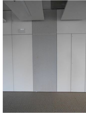
Figure 47 – Drilled wall panel to exhaust hot air (July 2015)
