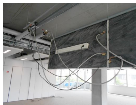
Figure 51 – Back side of heat/cold ceiling emitters with LED light (July 2015)
