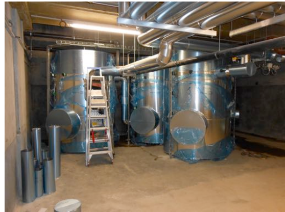
Figure 53 – Water tanks after full insulation (July 2015)
