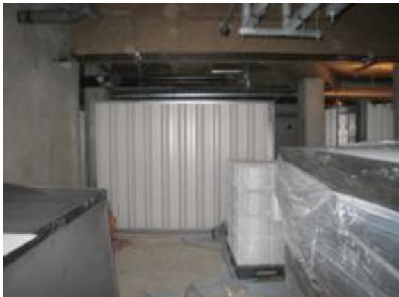
Figure 54 – PCM tank used as cold storage (December 2014)
