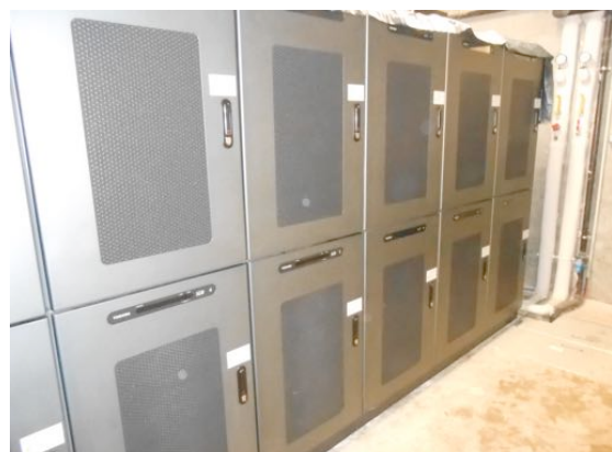
Figure 57 – Overview of the 100 kW hybrid battery (July 2015)
