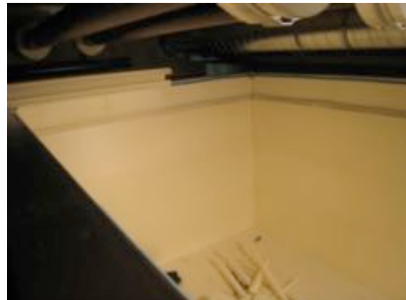
Figure 55 – Inside of the PCM tank before PCM installation (December 2014)
