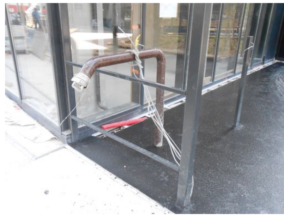
Figure 45 – Rapeseed oil filling pipe (July 2015)
