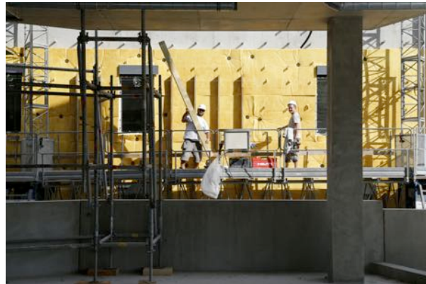
Figure 31 – Outdoor insulation of MINAMI (September 2014)
