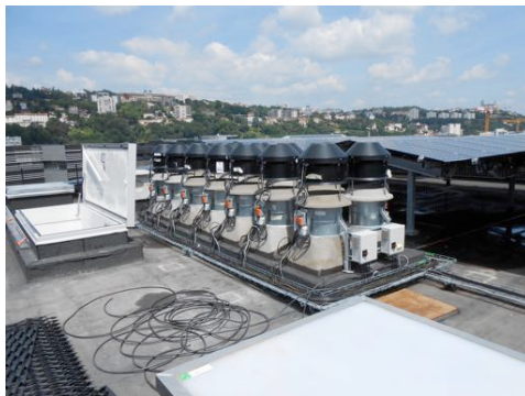
Figure 48 – Rooftop air outlets to control natural ventilation (July 2015)
