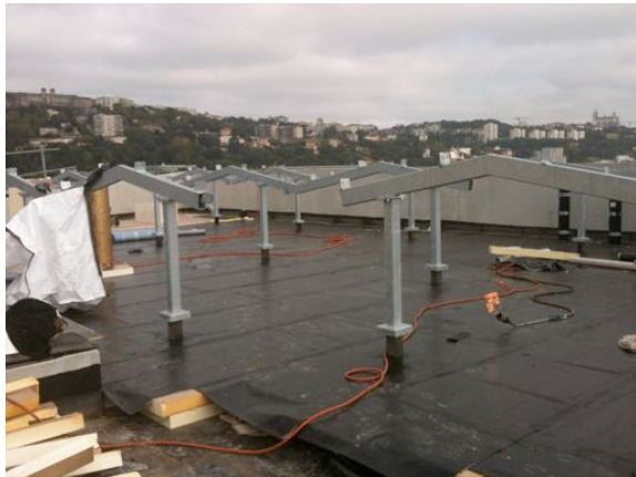
Figure 36 – Support structure of the rooftop PV system (November 2014)
