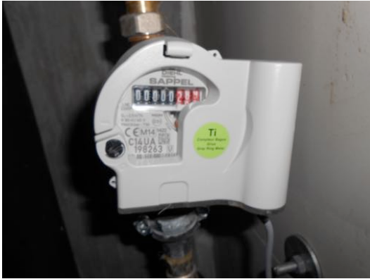
Figure 58 – Smart water meter that sends data to the HEMS (July 2015)
