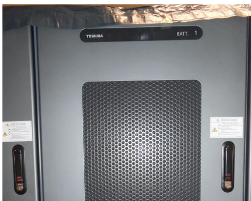
Figure 56 – Element of the 100 kW hybrid battery use for power storage (July 2015)
