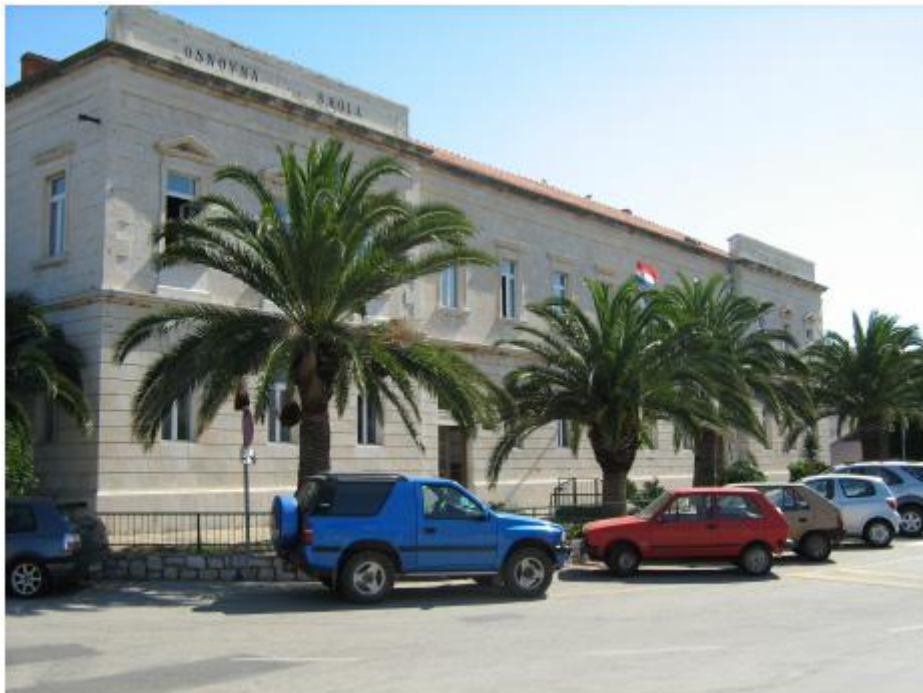
Figure 2 Typical historic building in Stari Grad
