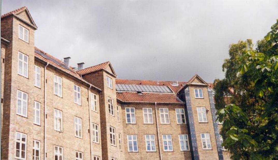
Fig. 3.1.1.5. Low energy retrofit housing at Lineagaarden, Frederiksberg in Copenhagen. PV is matching energy use in shared HRV systems for 200 housing units.
