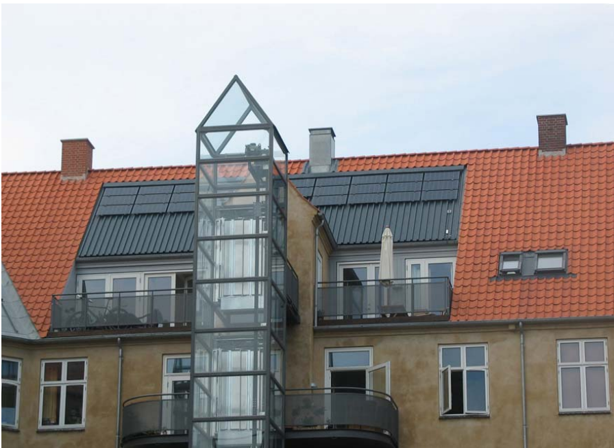
Fig. 3.1.1.6. Air solar collector with PV modules at Lauritz Sørensens Gård, Frederiksberg, Copenhagen. Ventilation air is here preheated before entering HRV systems.
