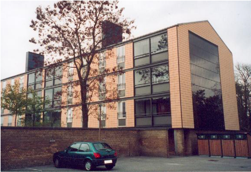
Fig. 3.1.1.7. Test of different types of HRV systems in combination with PV to match electricity use for ventilation at a low energy retrofit housing scheme in Lundebjerg, Skovlunde near Copenhagen.
