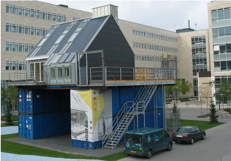
Fig. 1: CO 2 neutral rooftop apartment. Exhibition in Ørestaden, Copenhagen.
