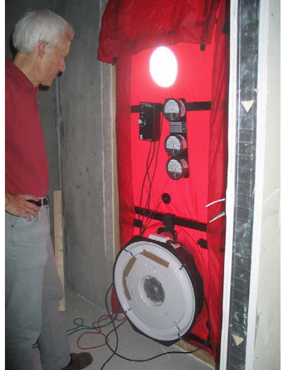
Fig. 2.6.1.3. Blower Door equipment with fan installed in one of the exterior doors of the building.
