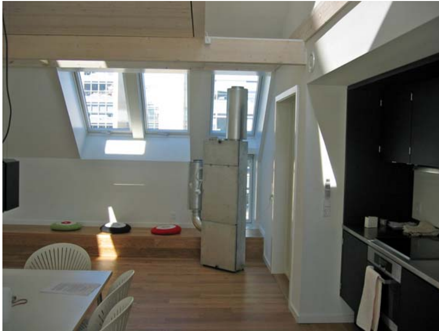
Fig. 3.1.1.1.: Illustration of an only 22 cm thick heat recovery ventilation unit which can be integrated in a partition wall or placed over a suspended ceiling, in both new build and retrofit housing projects.
