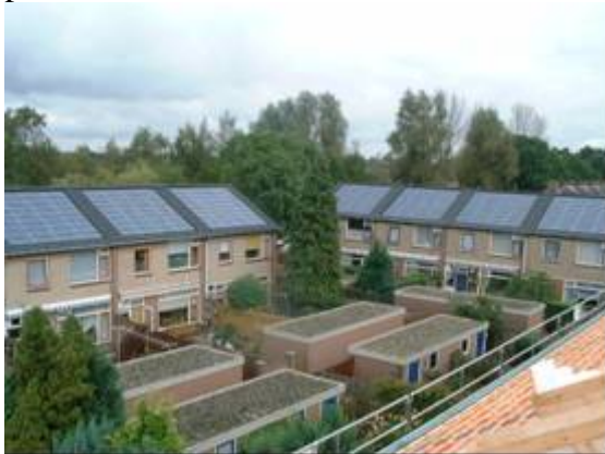
Figure 8. Renovation 364 dwellings in Apeldoorn: 1 MW project
