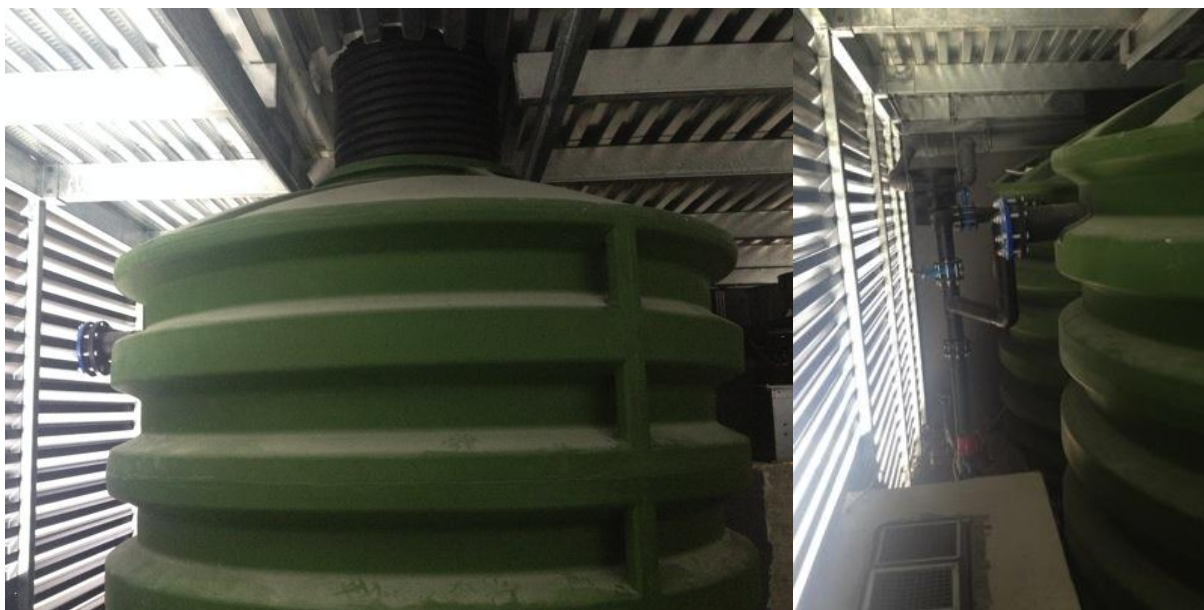
Picture 5: Rainwater storage tanks ESH
