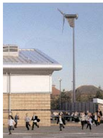
Fig 3.25 6 kW wind generator at Cumbernauld Primary School, Scotland.
