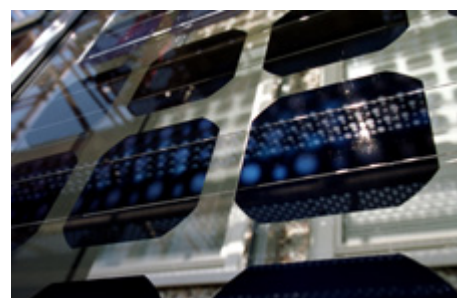
Fig. 3.24 Photovoltaic cells laminated into glass modules in the façade of a building at the University of Trondheim.
