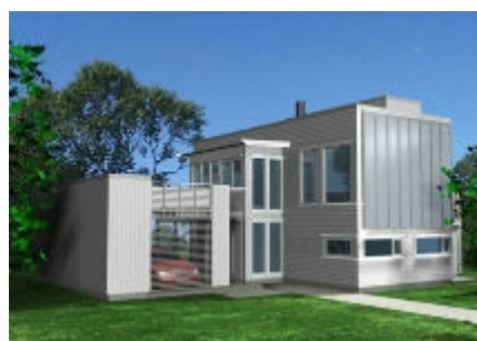
Fig. 3.10 Norwegian dwelling with flat-plate solar collectors on the façade. Source: www.systemhus.no
