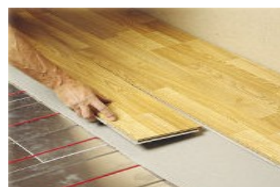
Fig. 3.2 Electric floor heating system with cables for wooden floor
