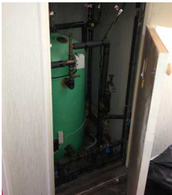
Figure 4: storage tank connected to condensing gas boiler from 2000 – 2014. (Picture Chiel Boonstra, Trecodome)
