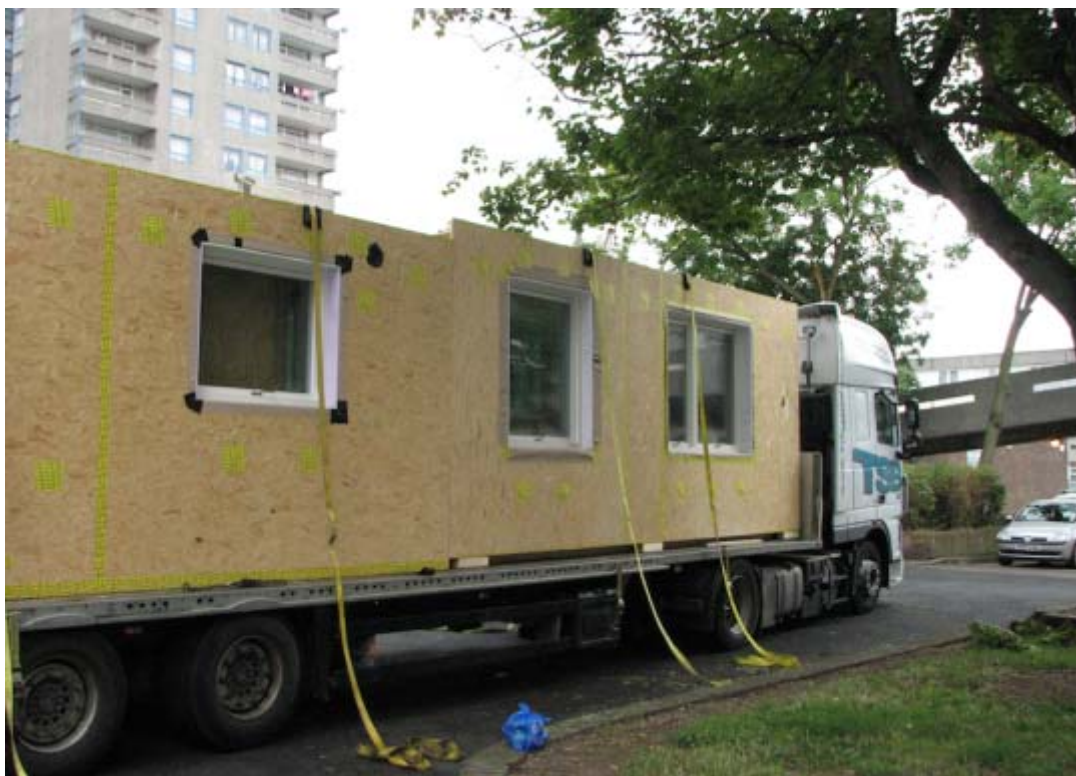
Figure 12: Arrival of the prefabricated TES façade elements from Germany at Parkview Hub. (Picture Martin Montgomery, Gump & Maier UK Ltd.)
