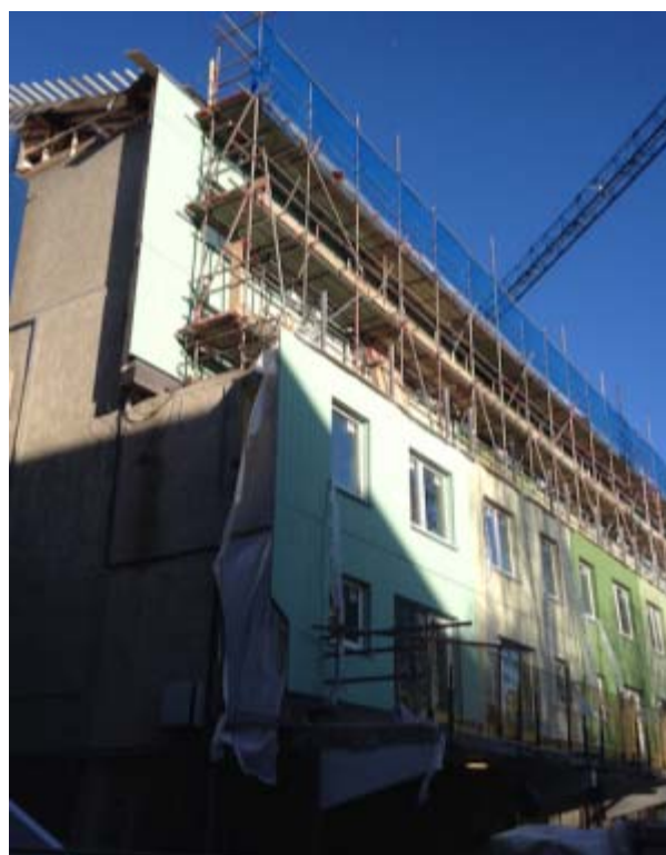
Figure 18: The final end façade can be installed once the staircase at the other side is completed. (Picture Chiel Boonstra, Trecodome)
