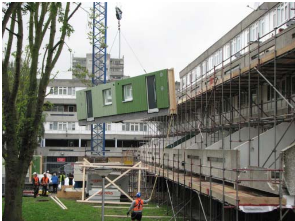
Figure 14: The elements are craned to other side of the building. (Picture Martin Montgomery, Gump & Maier UK Ltd.)
