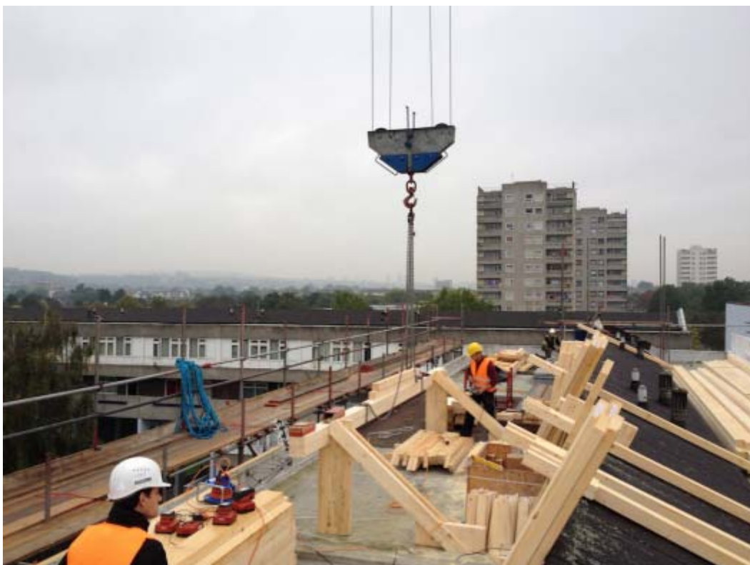
Figure 16: The new pitch roof construction on top of the existing flat roof. (Picture Chiel Boonstra, Trecodome)
