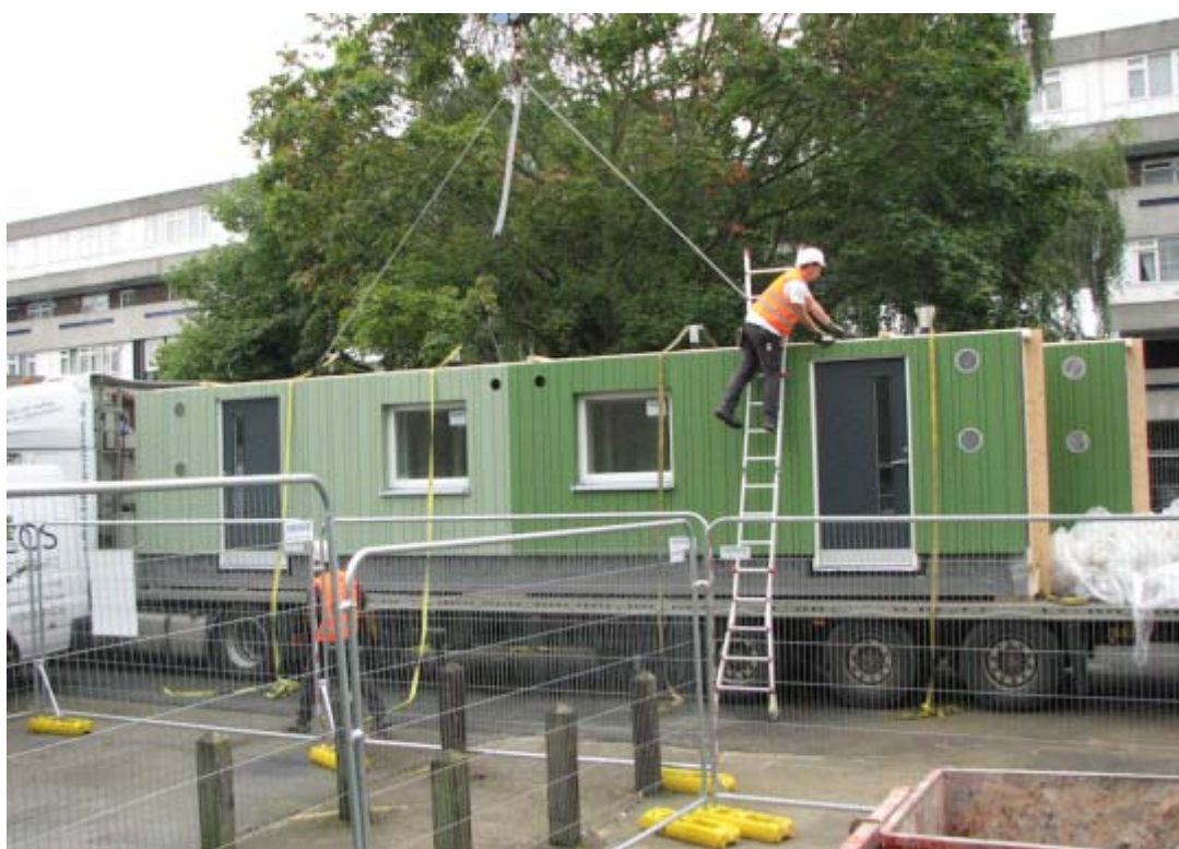
Figure 13: Mounting of the façade elements at the North facing façade. (Picture Martin Montgomery, Gump & Maier UK Ltd.)
