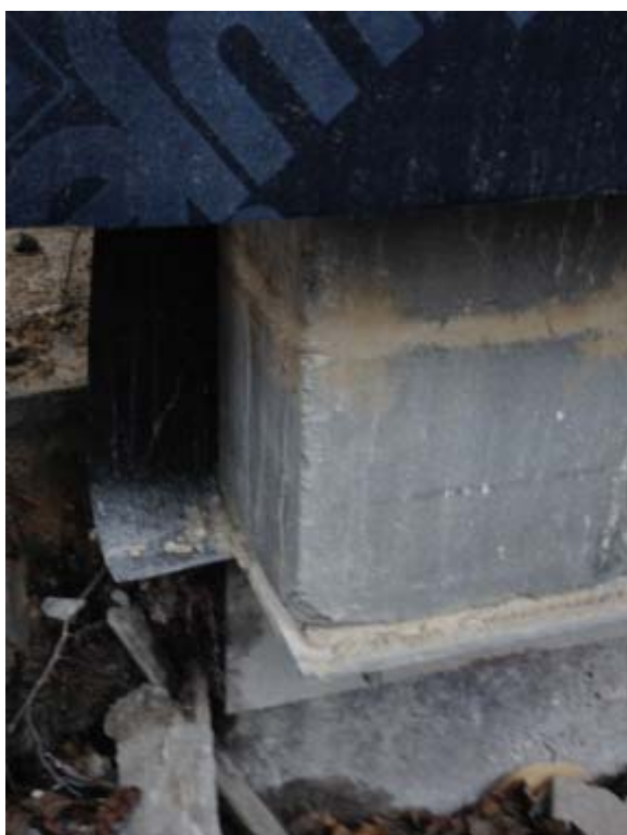
Figure 17: Foundation detail for the end façade with cellular concrete on a steel profile with the prefab element on top. (Picture Chiel Boonstra, Trecodome)
