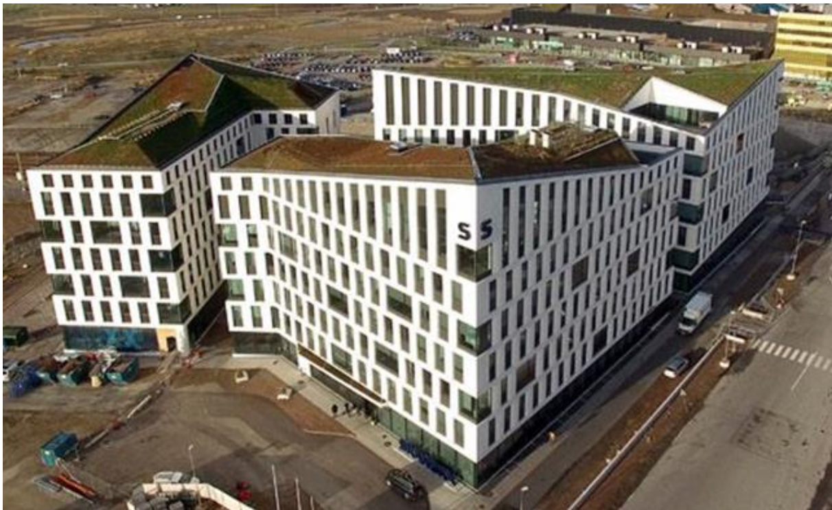
Figure 6 The office building Klipporna [9].
