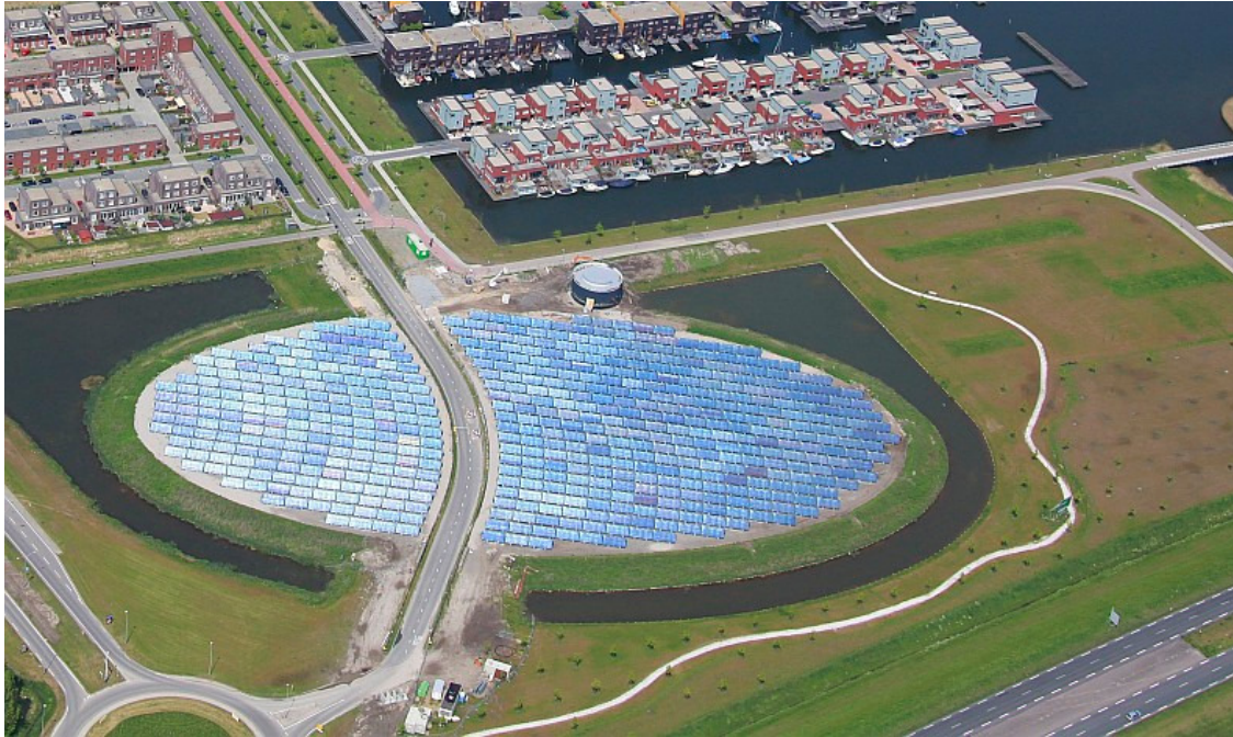
Figure 8- An aerial photo of the Solar Island during construction. Courtesy of Nuon
