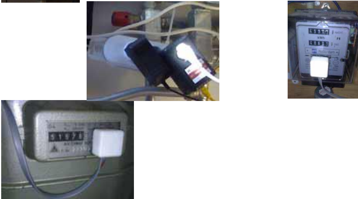
Figures 4-6: Connection to wireless communication for sensors metering electricity and gas.
