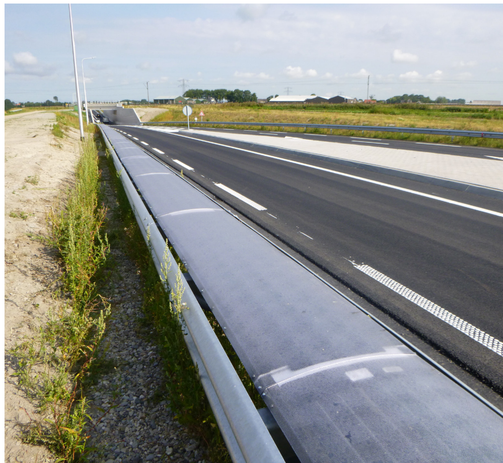
PV integration in 72 m long double guardrail along the N194 near Heerhugowaard, the Netherlands. ©Solliance | solliance.eu
