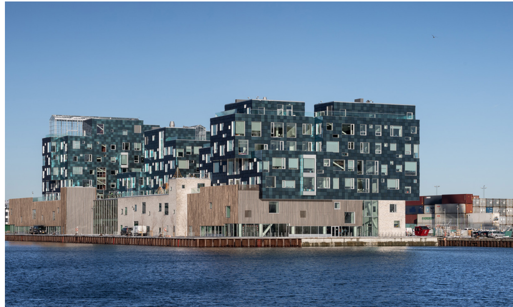
©Adam Mørk. Copenhagen International School building with 12 000 square-shaped, coloured BIPV panels.
