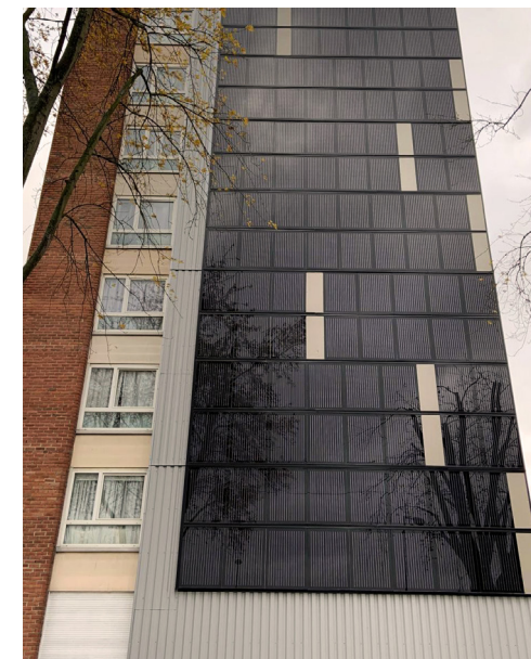
BIPV ventilated façade of apartments building, Wattignies, France. ©Onyx | onyxsolar.com PV Sites demonstration project.
