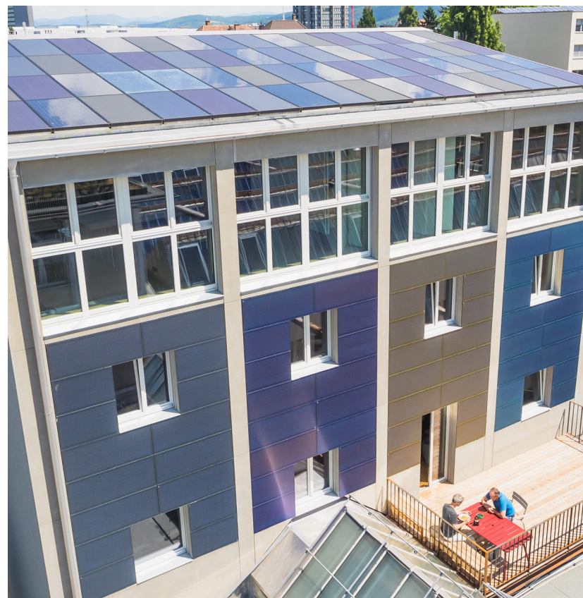
Reconstruction of historic building with coloured BIPV. ©Argola Solvatec, SolarSilo Basel 2015.
