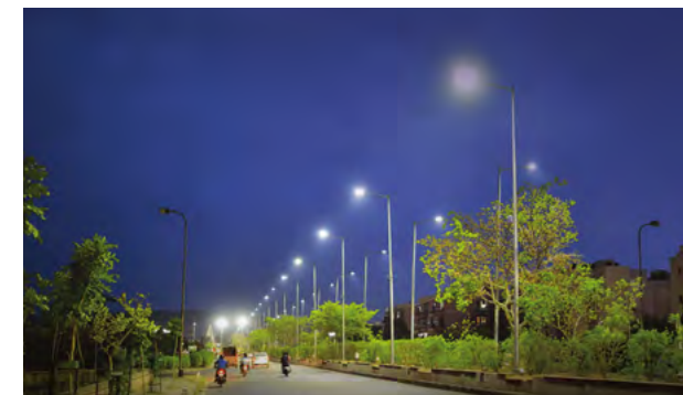
In Jaipur, India, smart streetlights with motion sensors and wireless controllers adjust brightness in real-time based on human presence, enhancing city services and safety. © tvilight.com
