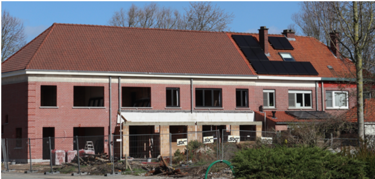
↑ Retrofitting an insulation works in Kortrijk, Belgium. © Agata Smok
