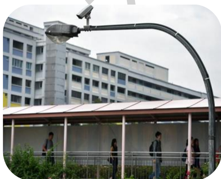
Lamppost retrofit Adding new things into a existing asset
