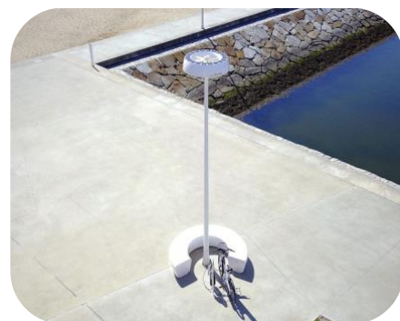
Multi-functional pole Installing new smart integrated poles
