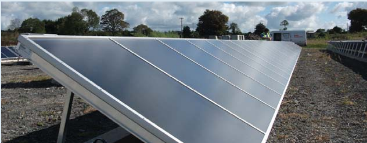
Eco-village Solar Park
