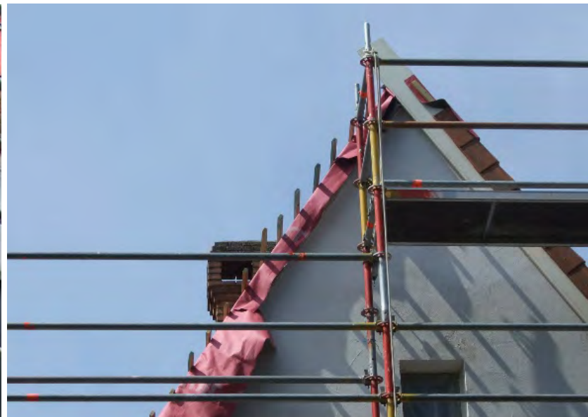
Illustration of need to redesign building nodes, e.g. where retrofitted roof and facade meet.
