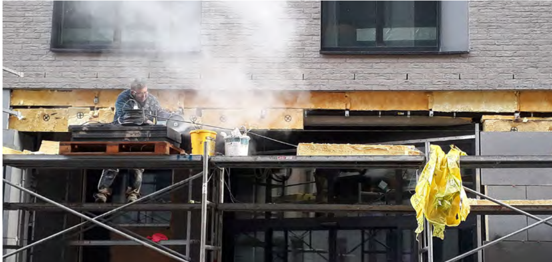
Doing a bad job: when the insulation panels do not connect well and tightly to each other, much of the insulation capacity is lost. Capacity building in the work force and strict control of the building works are essential to avoid such situations.
