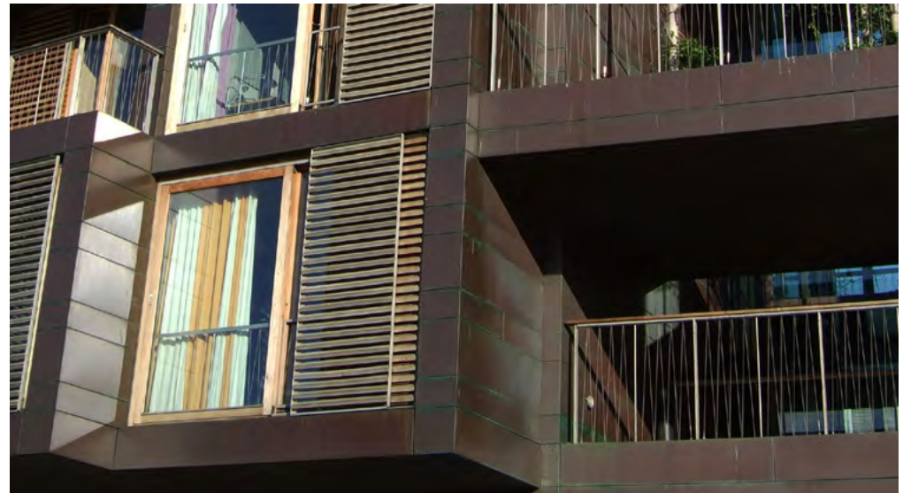
External shading integrated in the architecture of the building: overhangs, mobile louvers (Tietgenkollegiet, Copenhagen)
