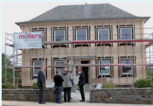
Image 3.3: Retrofitting of the Old Presbytery, Redange (LU)
