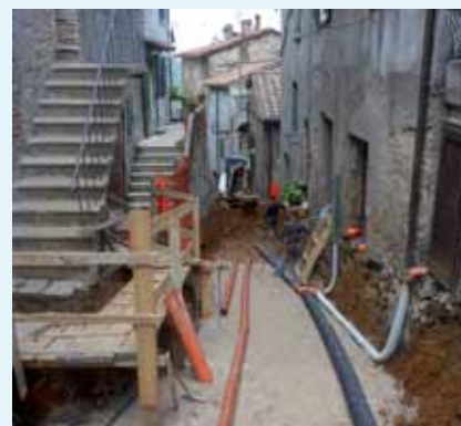
Image 3.6: Installing Geothermal District Heating in the Historic Centre of Montieri (IT)
