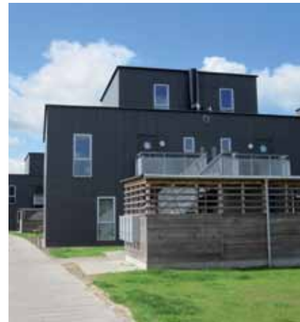
Image 2.4: Ultra-low Energy Houses in Stenløse (DK)
